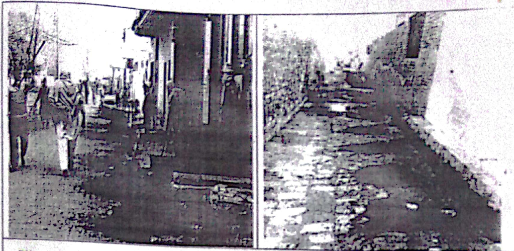
Silt and muck is taken out from drains, semi dried and collected in the loader rikshaws
