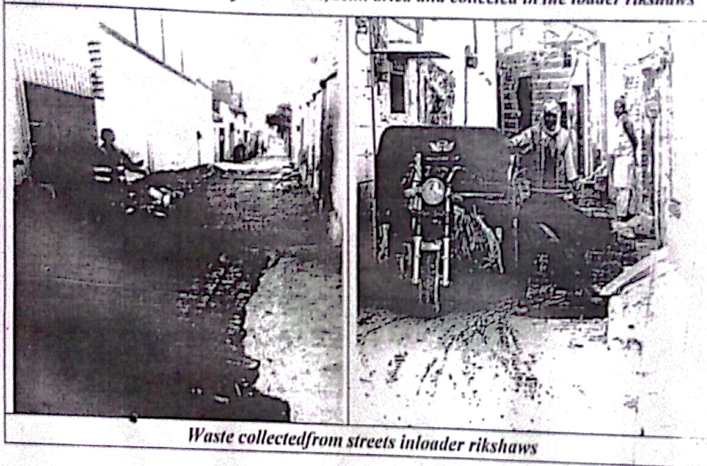
Silt and muck is taken out from drains, semi dried and collected in the loader rikshaws
