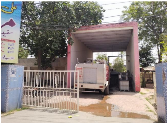
Figure 31: Front view of Fire Brigade
