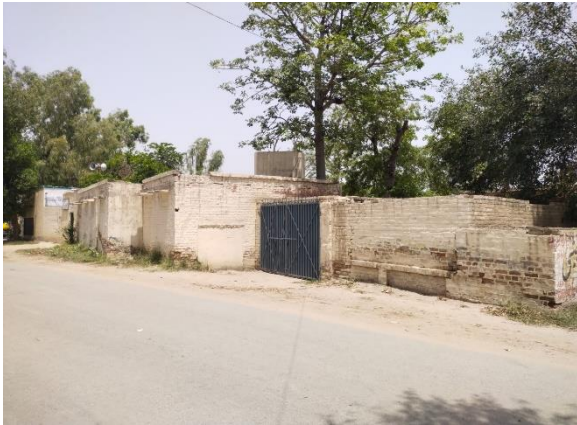
Figure 25: Front view of Camp office & residency
