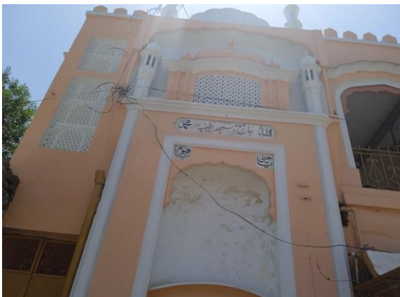
Figure 20: Front view of MC Mosque
