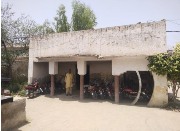
Figure 27: Front view of Library & Quarter & Workshop
