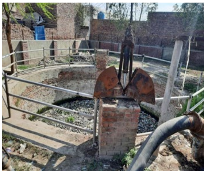
Figure 4-20 Cleaning of wet well with clamshell excavator
