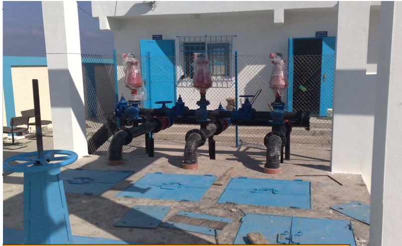
Figure 4-7 Force main and header
