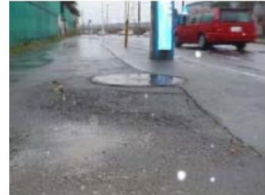
manhole damaged
