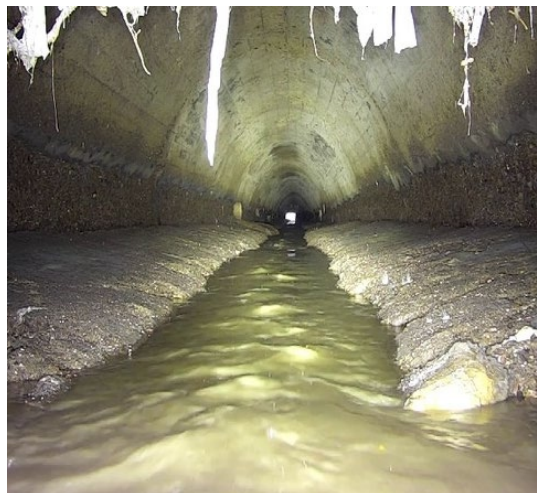
Figure 2-2 Sewer inspection with camera
