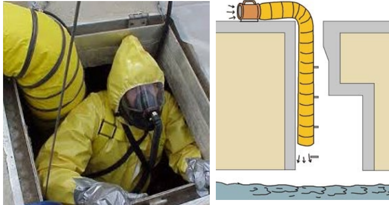
Figure 3-6 Fresh air should be supplied to the working location and the blower fan must be carefully located to avoid sucking in contaminated air.
