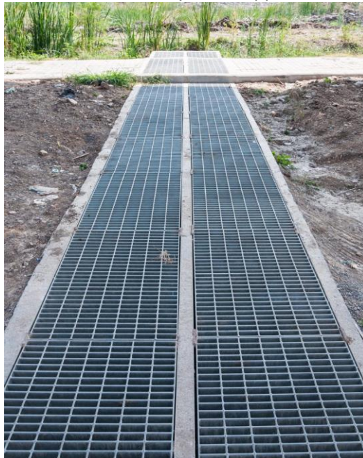
Figure 16: Trench drain
