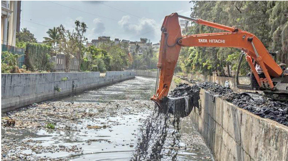
Figure 79: Routine drain cleaning
