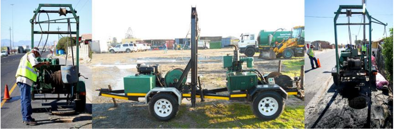
Figure 82: Cleaning of closed drains using a bucket
