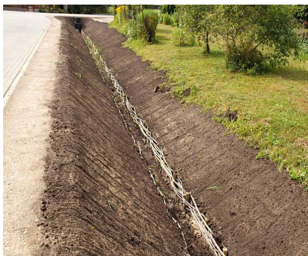
Figure 128: Side slope erosion can cause rollovers
