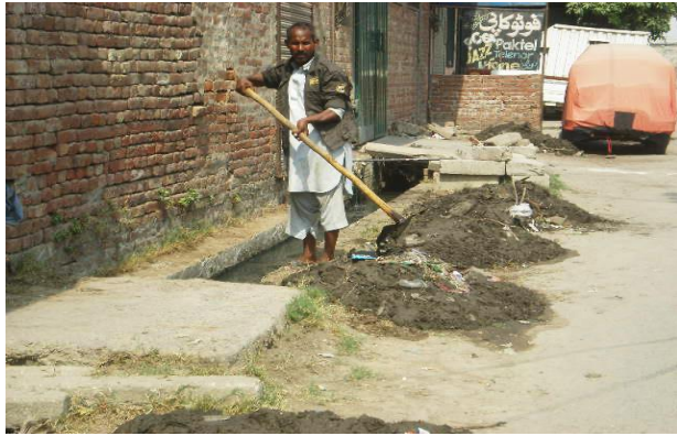
Figure 80: Manual Desilting
