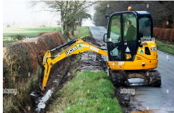
Figure 81: Mechanical Desilting
