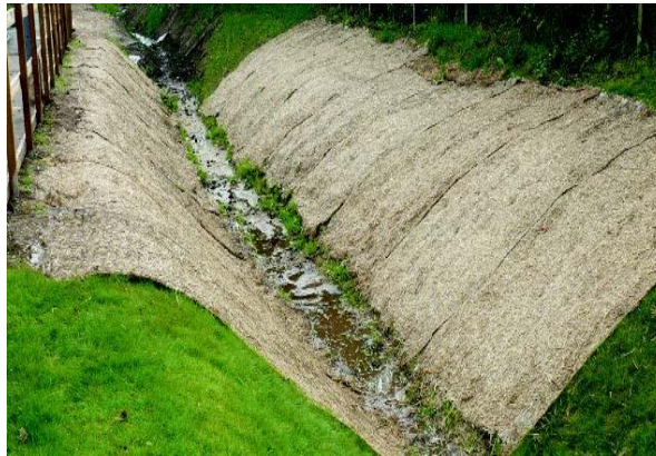
Figure 101: Soil Retention Blanket application on slopes
