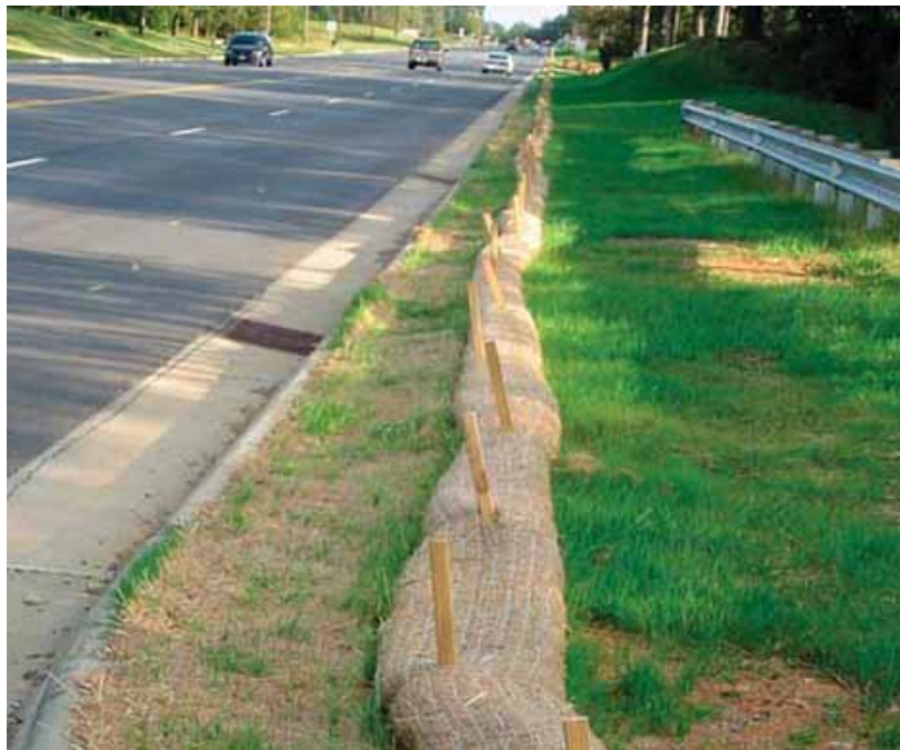
Figure 107: Slope breaks
