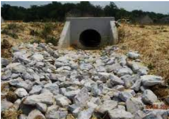
Figure 32: Storm drain outlet channel 1
