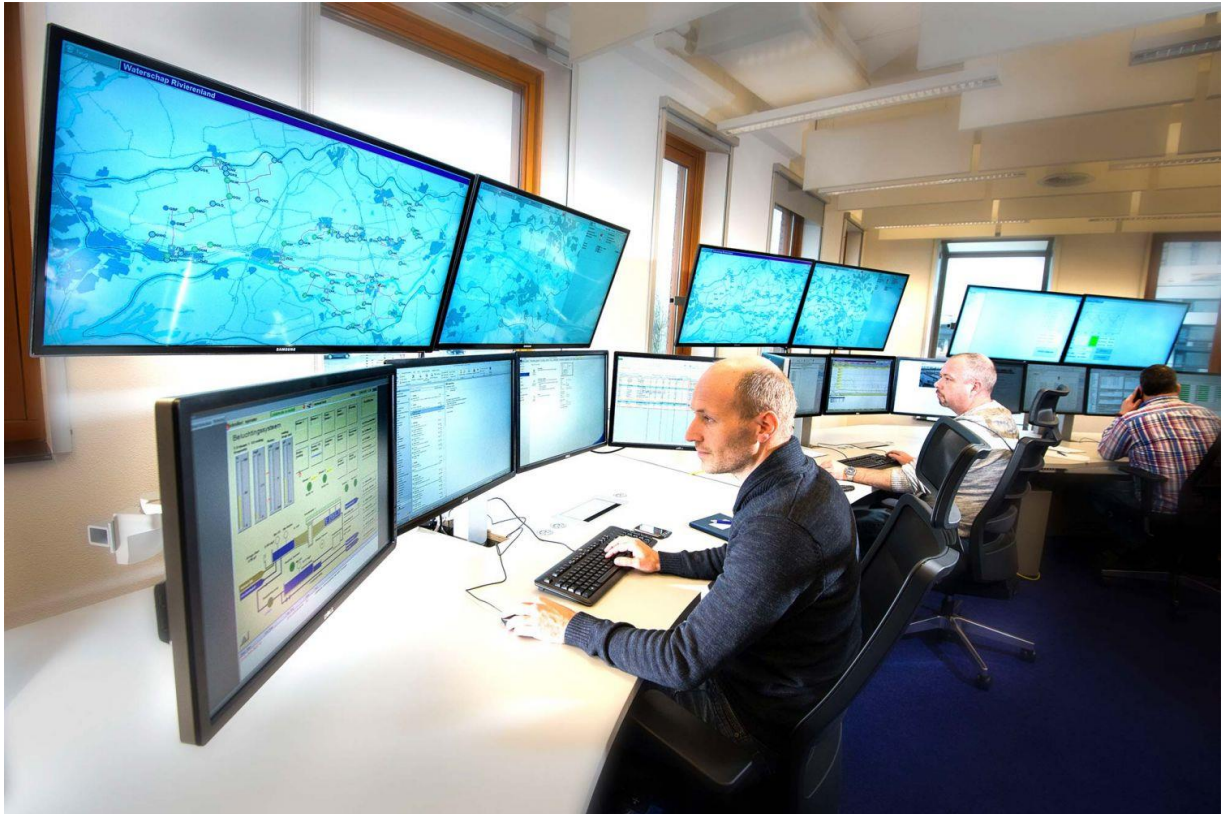
Figure 40: Storm control Room
