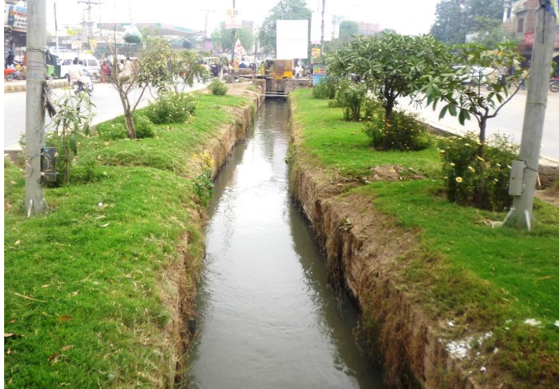
Figure 74: Road connected with drain at proper slope through small drains
