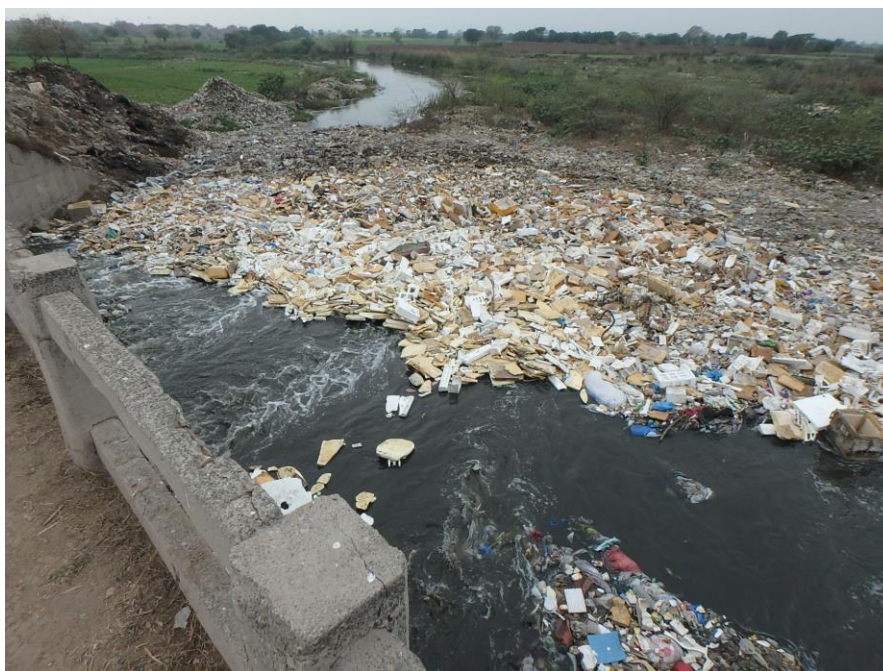
Figure 12: Transportation of wastewater in open drain
