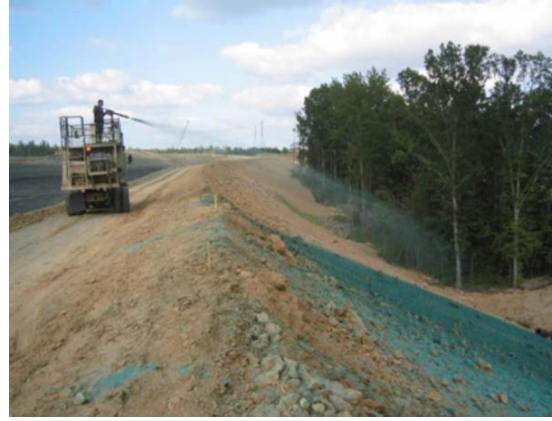
Figure 100: Mulching on disturbed surface
