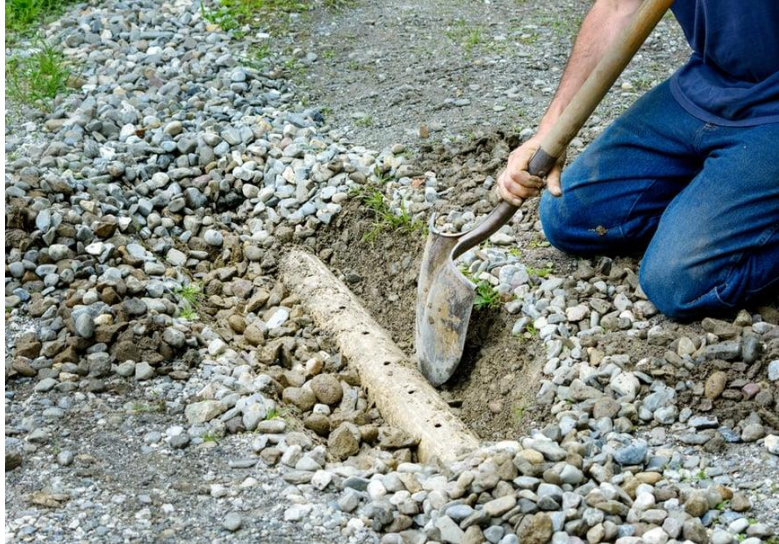
Figure 15: French drain
