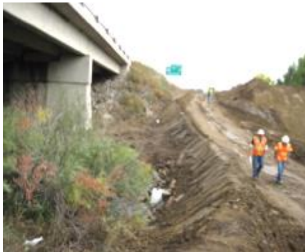
Figure 103: Temporary Berm along access road
