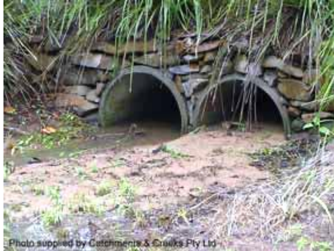
Figure 36: Blockage of stormwater pipes & culverts due to dust
