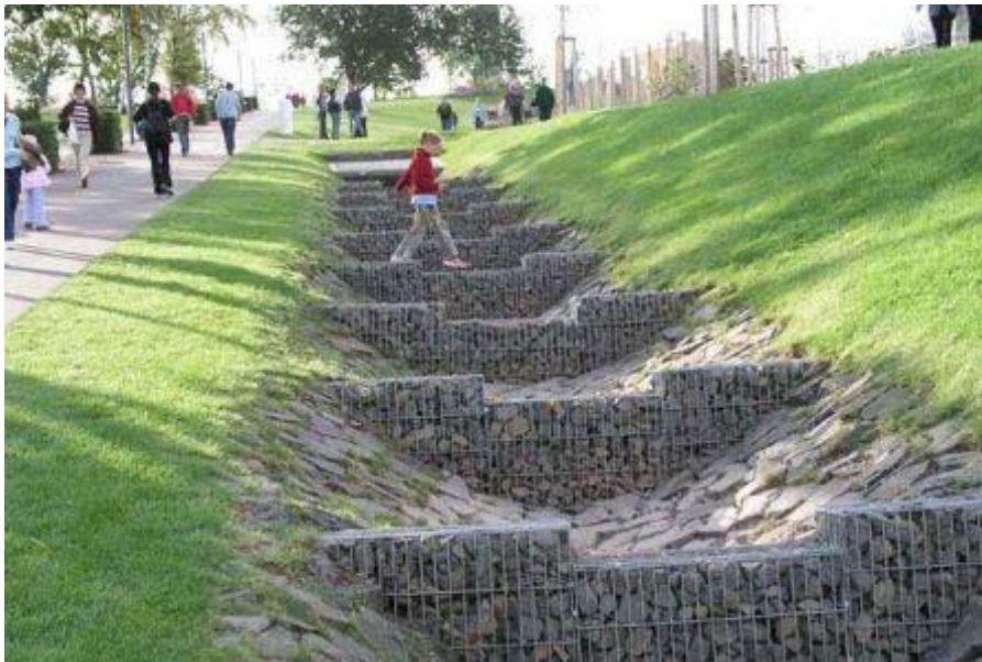
Figure 68: Baffles at a steep drain
