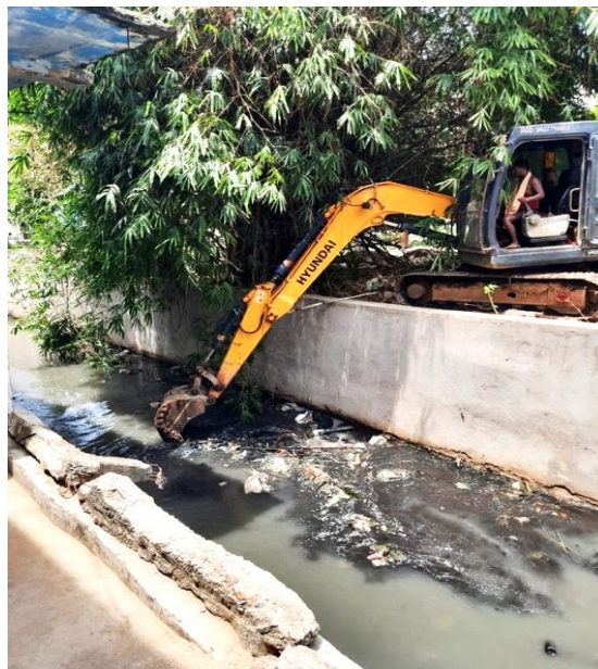
Figure 75: Desilting activity
