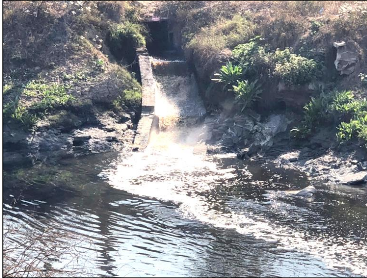
Figure 63: Effluent of an industry discharging directly into Drain
