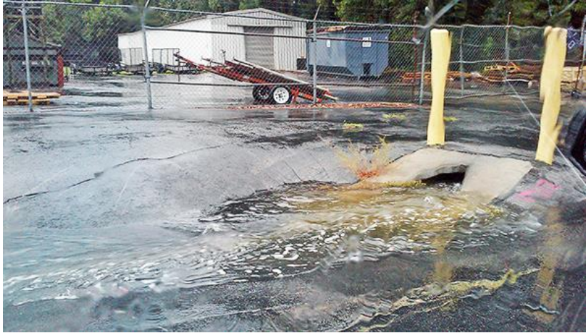
Figure 71: Water pressure in a closed drain
