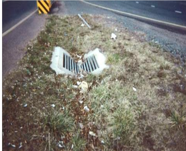
Figure 131: V-shaped grate in median.
