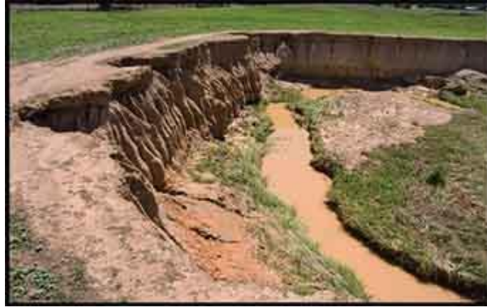
Figure 39: Erosion of a depressive soil
