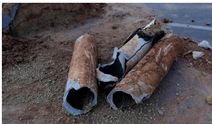
Figure 117: A damaged Sewage Pipe
