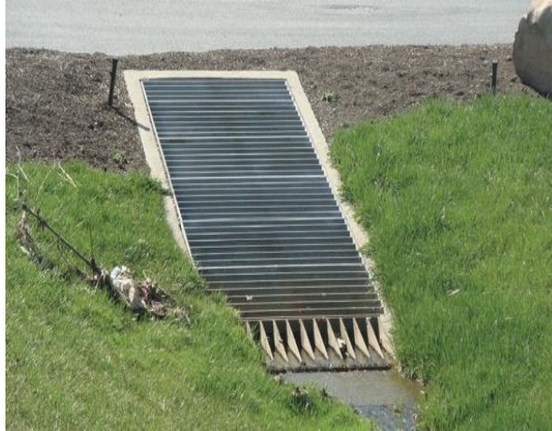
Figure 133: Grated inlet flush with ground over a culvert end
