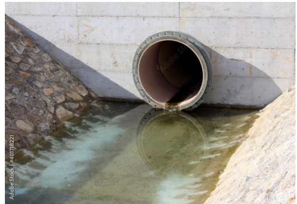
Figure 33: Storm drain outlet channel 2
