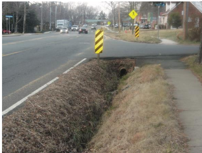
Figure 130: A non-traversable drainage ditch
