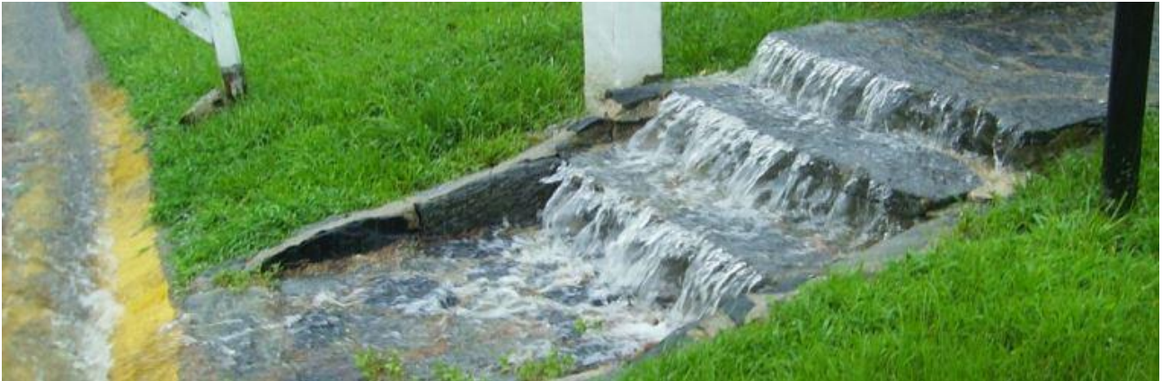
Figure 69: Steps at a steep drain
