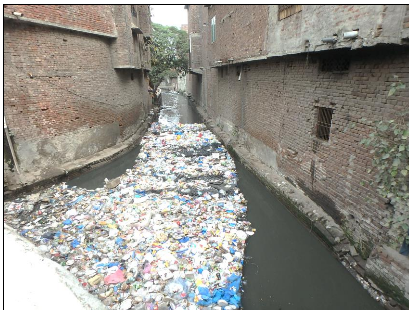
Figure 76: Encroachment at the banks of the drain
