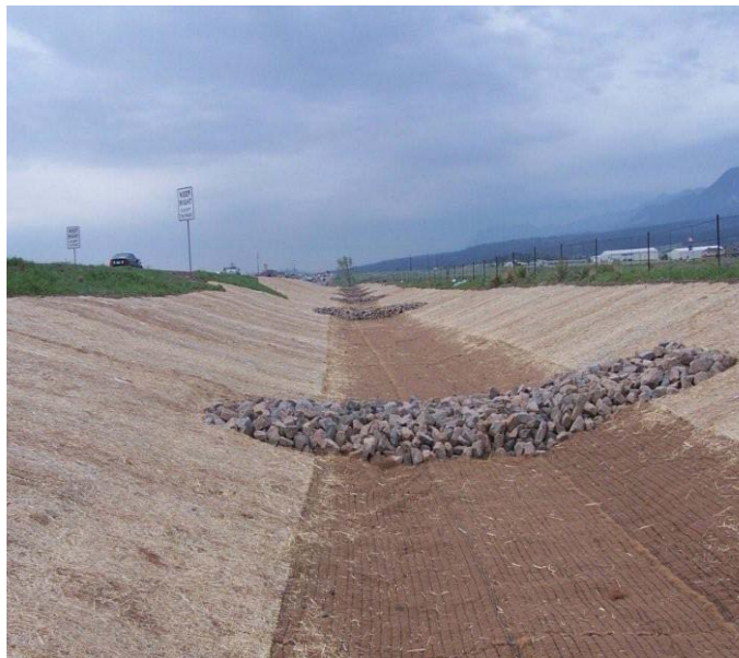
Figure 98: Rock check dam along lined drainage ditch
