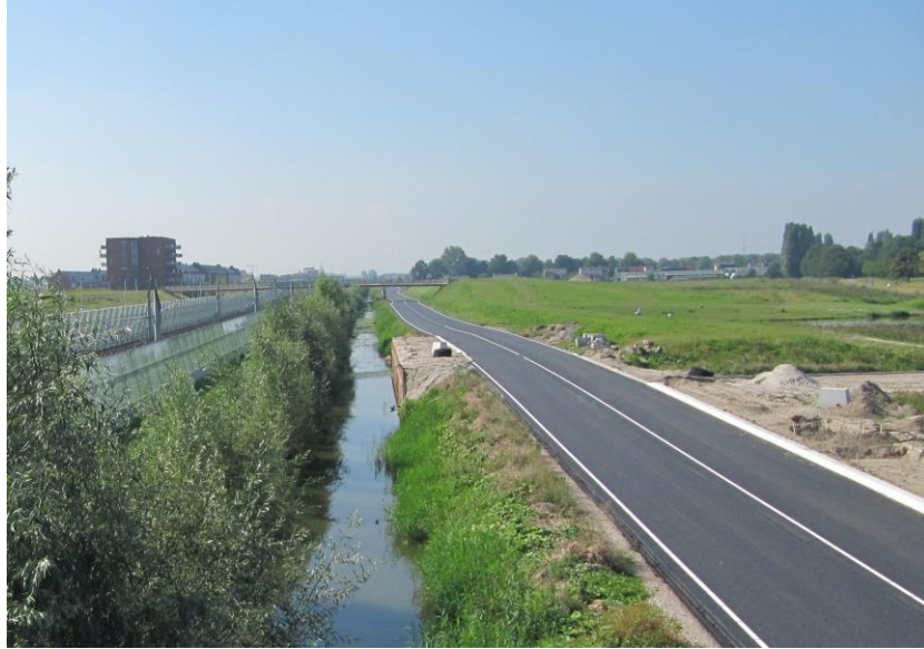
Figure 13: Open storm drain
