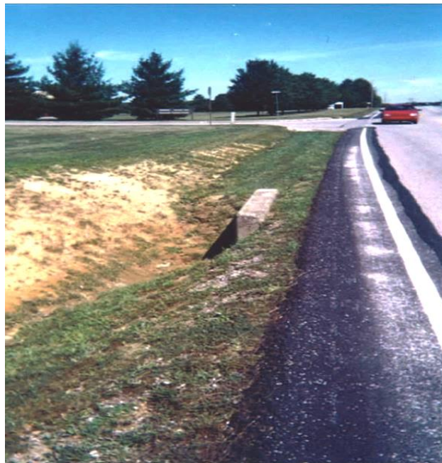
Figure 132: Culvert headwall is a roadside hazard
