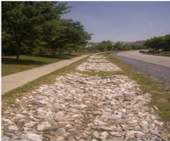
Figure 23: Infiltration Trench Type 1
