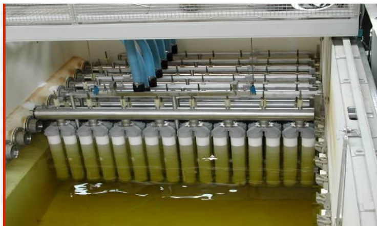
Figure 2-13: Membranes inserted in to sewage
