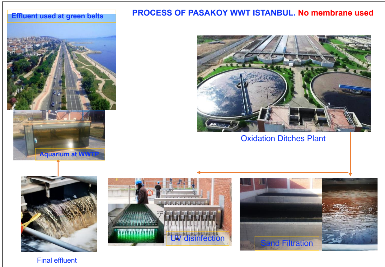
Figure 8-12: Treatment Process used at Pashakoy Istanbul
